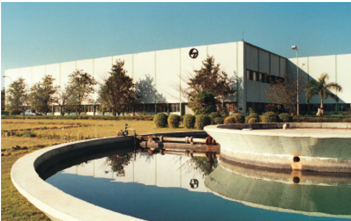
Switchgear Factory, Ahmednagar
