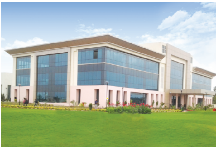
Switchgear Factory, Vadodara
