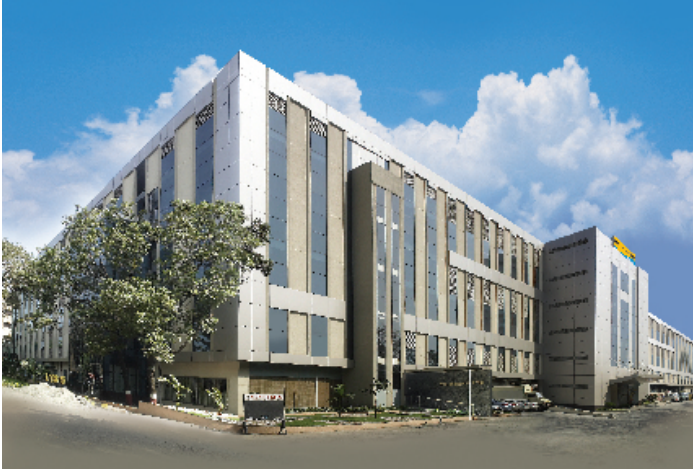
Switchgear Factory, Mumbai
